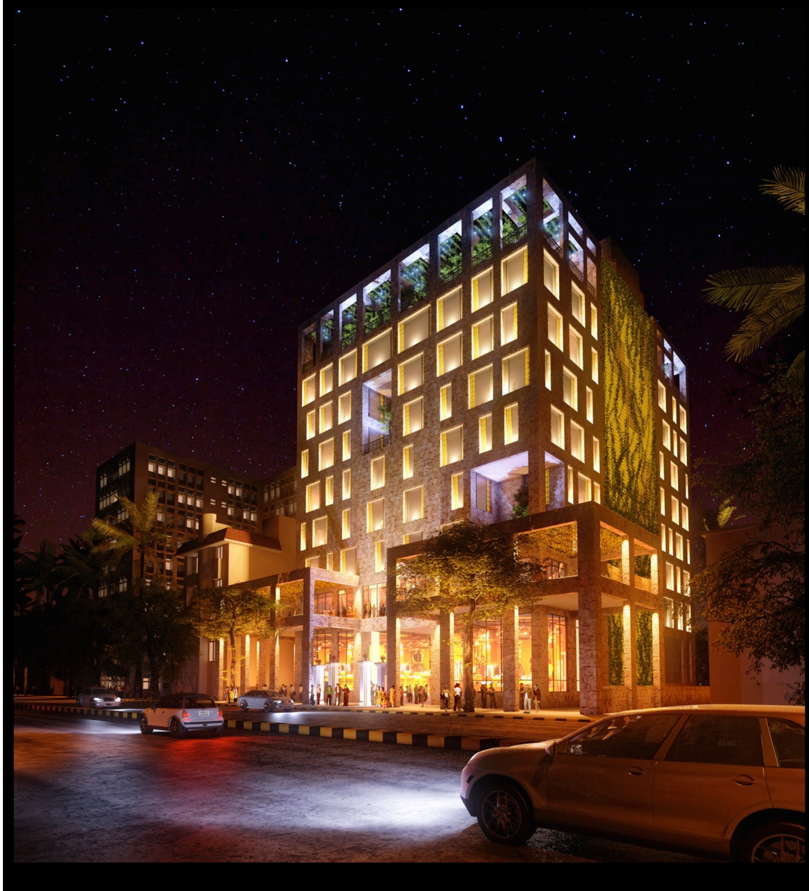
Office Building, Calcutta, India
